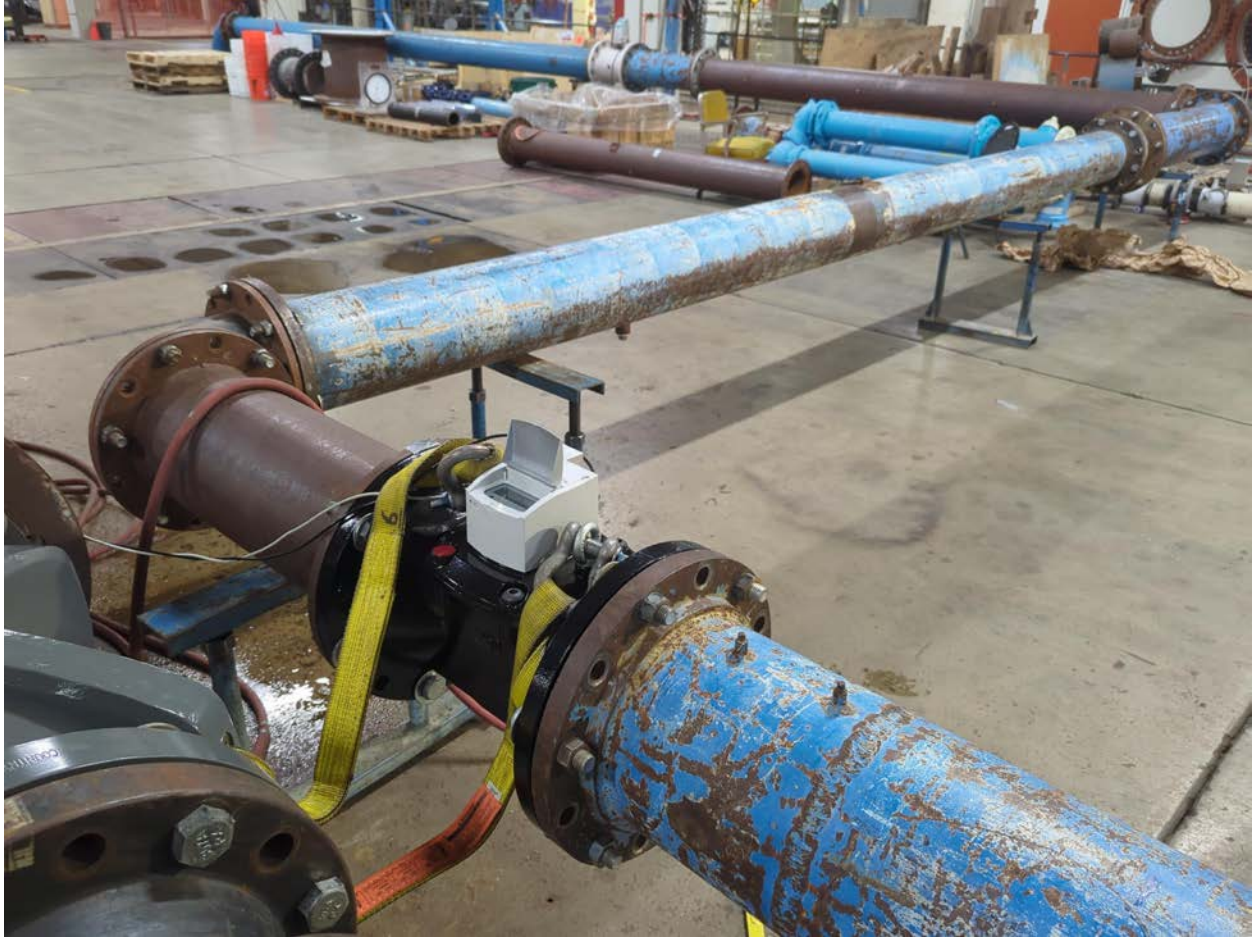
Figure 2 – Pipe Setup for 3D Elbow Test (flow goes left to right)
