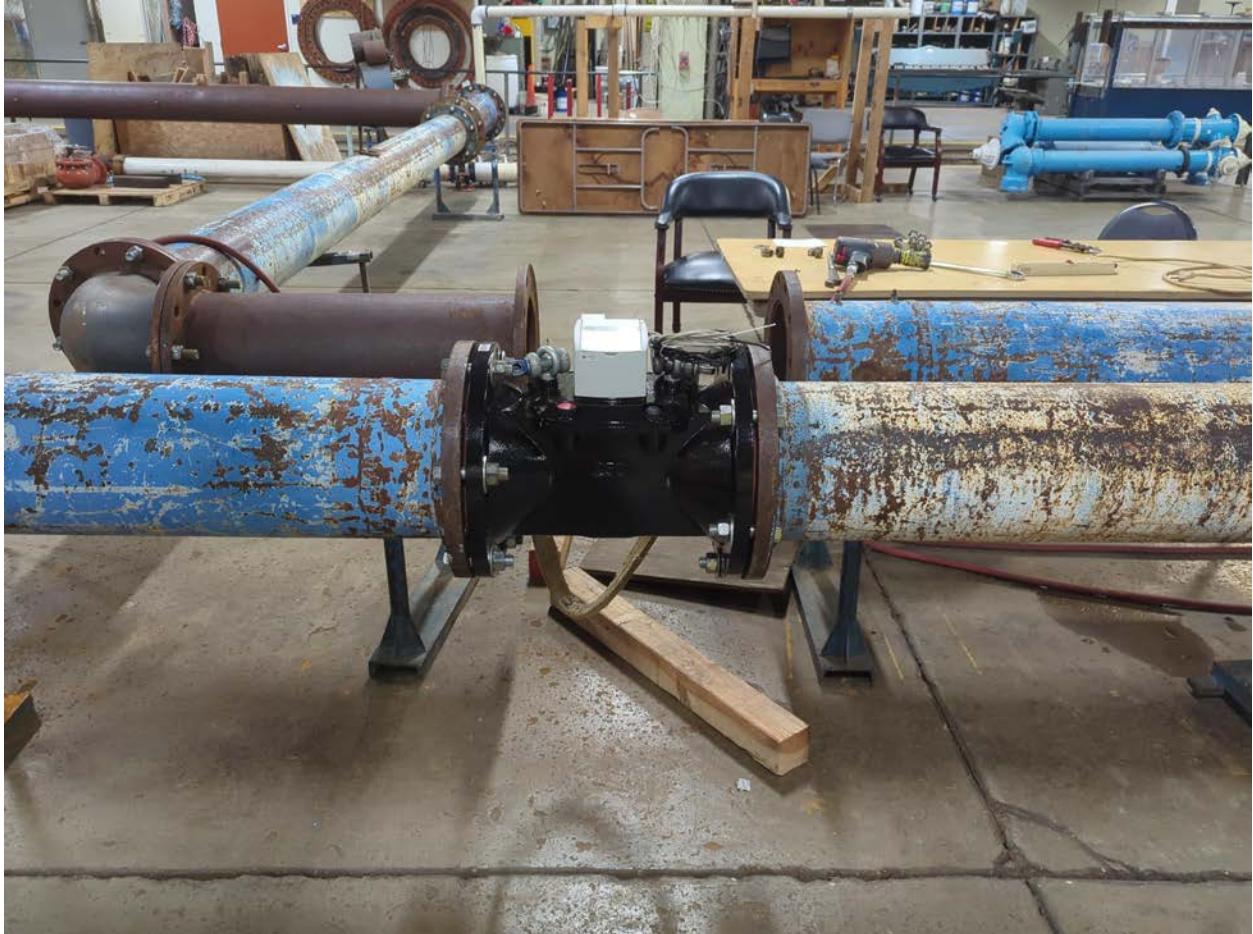
Figure 1 – Pipe Setup for Straight Pipe Test (flow goes left to right)
